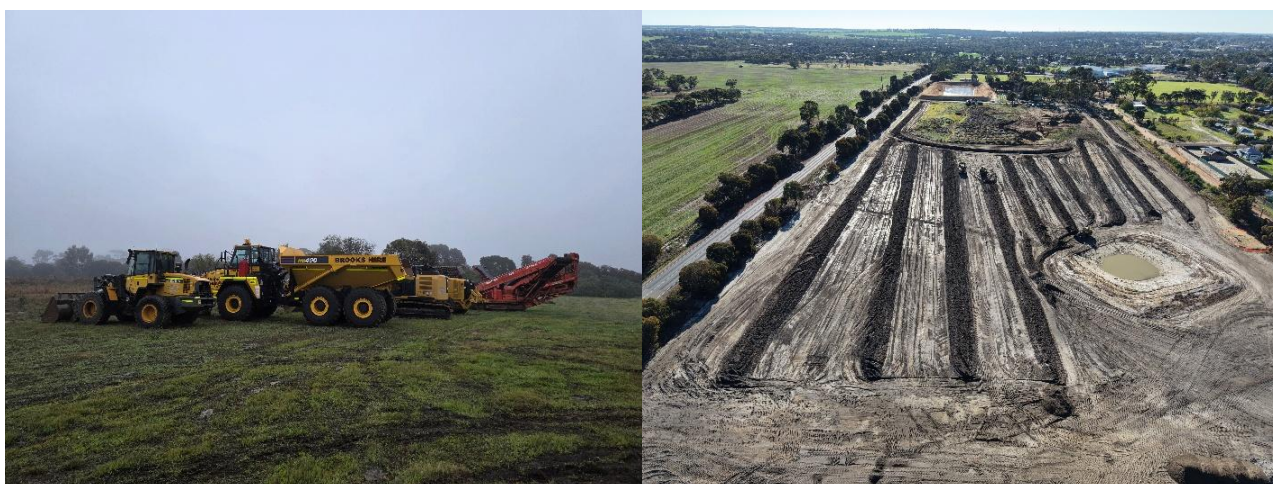
Equipment onsite at the Workforce Accommodation Village in Katanning (left) and land clearing underway (right).
