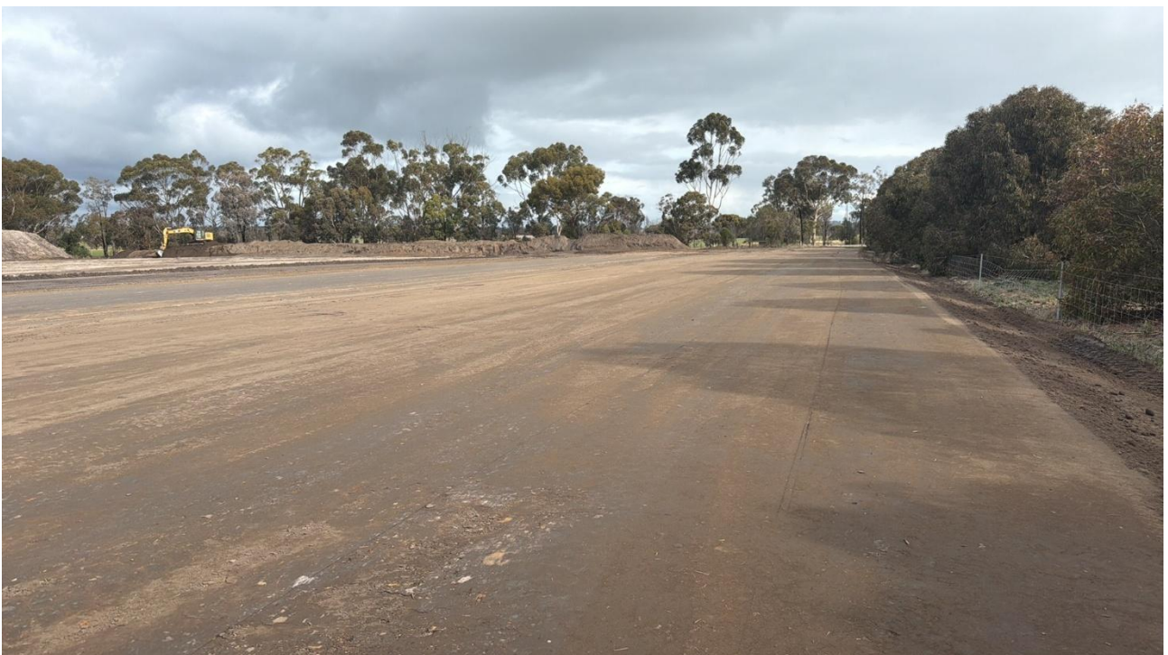
Workforce Accommodation Village site preparation well underway.
