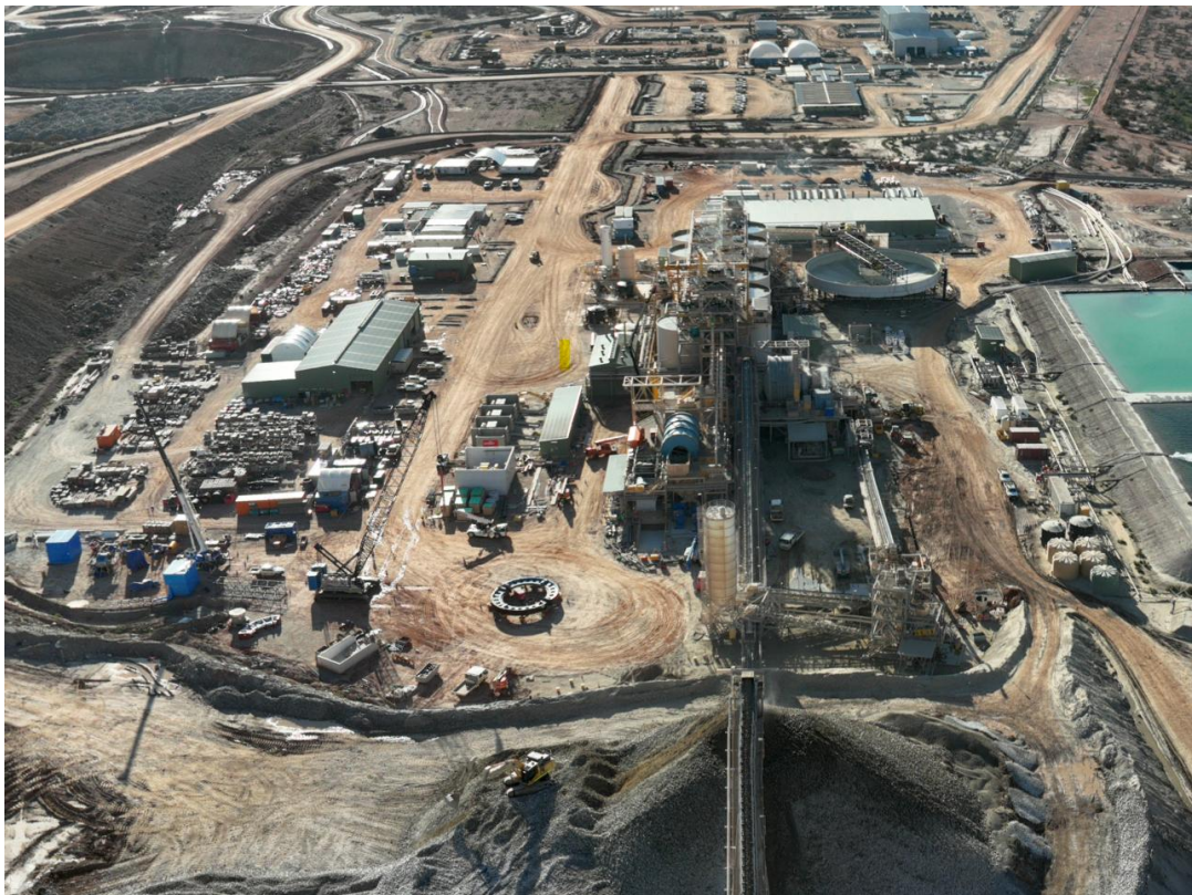
Figure 2: KoTH processing facility
