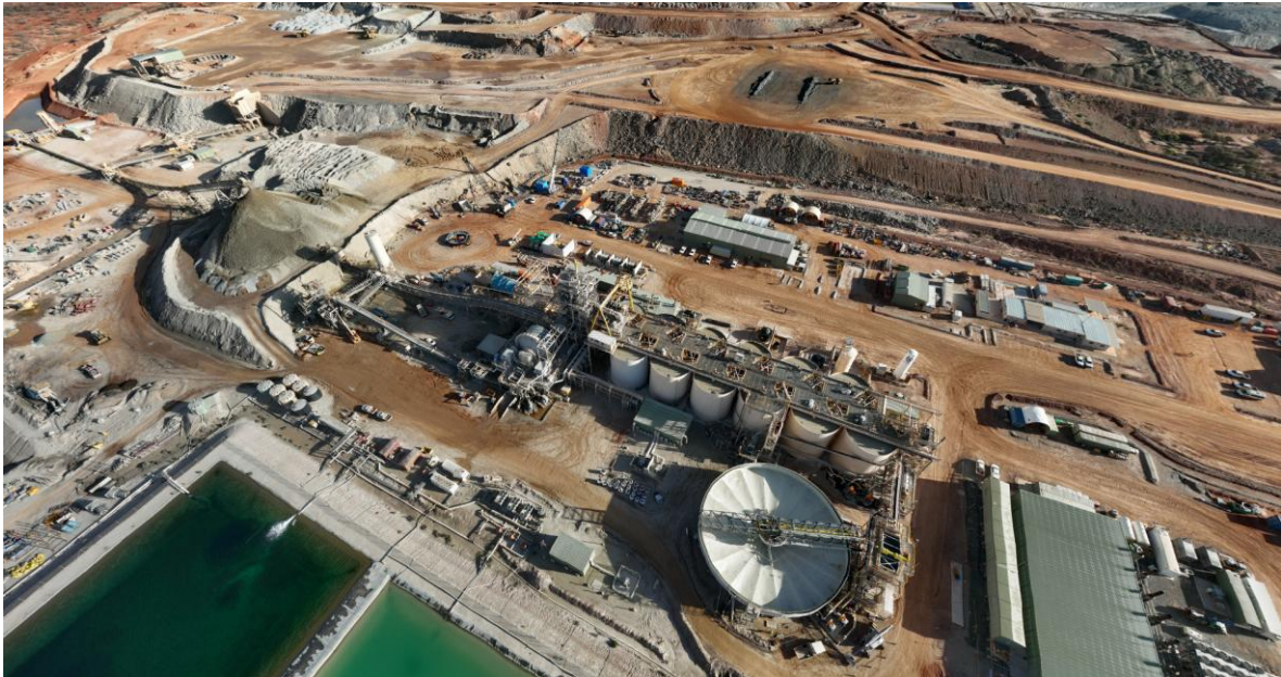
Figure 1: KoTH processing facility
