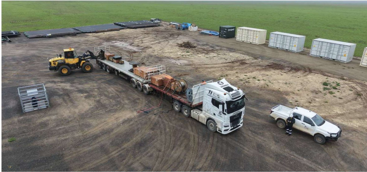
Figure 2: Mobilisation of equipment at the Ramsay Project in preparation for the upcoming flow testing campaign
