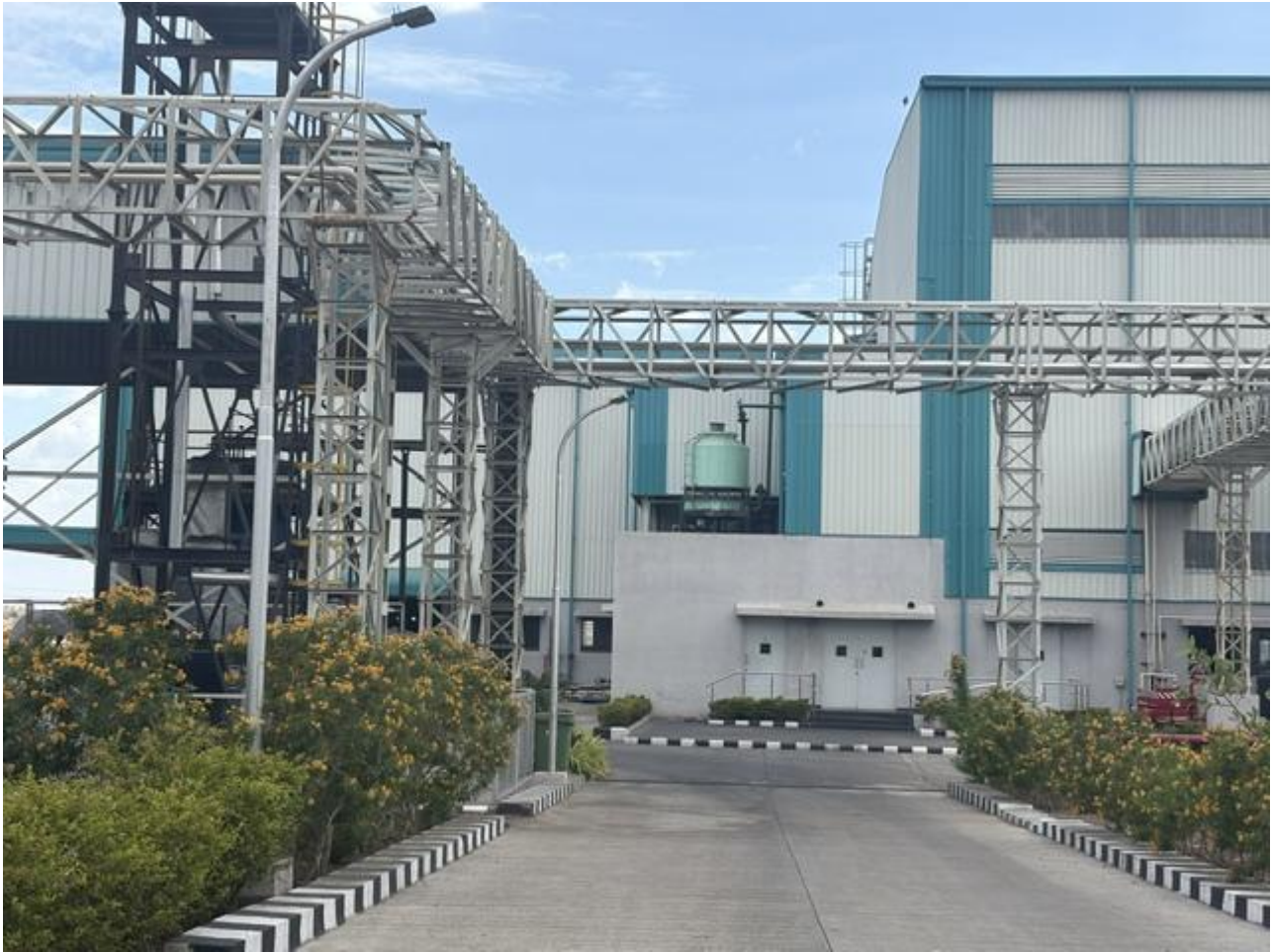
Figure 4 –PGT’s world leading production facility in India, June 2026
