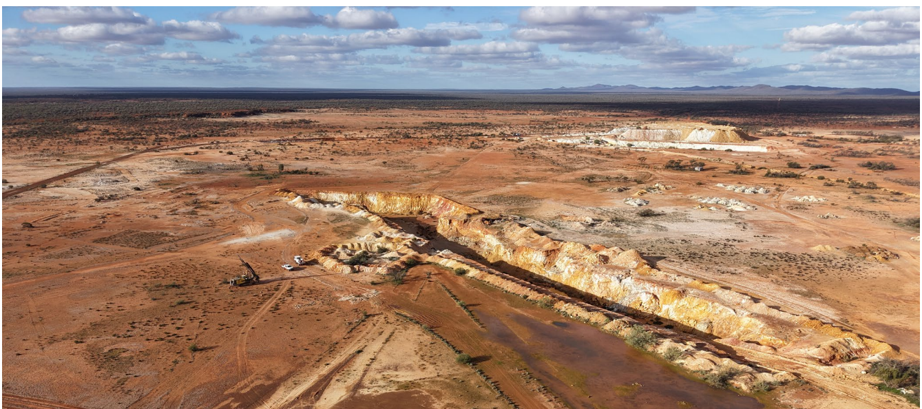
Figure 1. RC rig drilling underneath adjacent Mindoolah Main Reef old workings.
