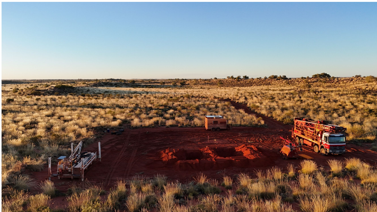
Figure 1: Madman Project, June 29, 2026. The McKay's rig onsite at the P1 drill pad.
