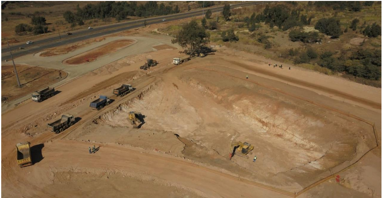
IMAGE 2: TERRACING WORKS ON THE POLLUTION CONTROL DAM
