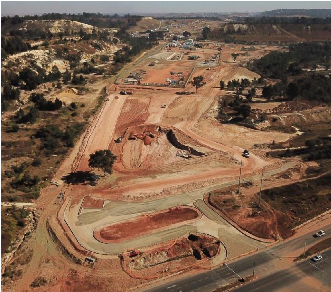
IMAGE 4: MAIN ENTRANCE ROADWAY, TERRACING AND POLLUTION CONTROL DAM
