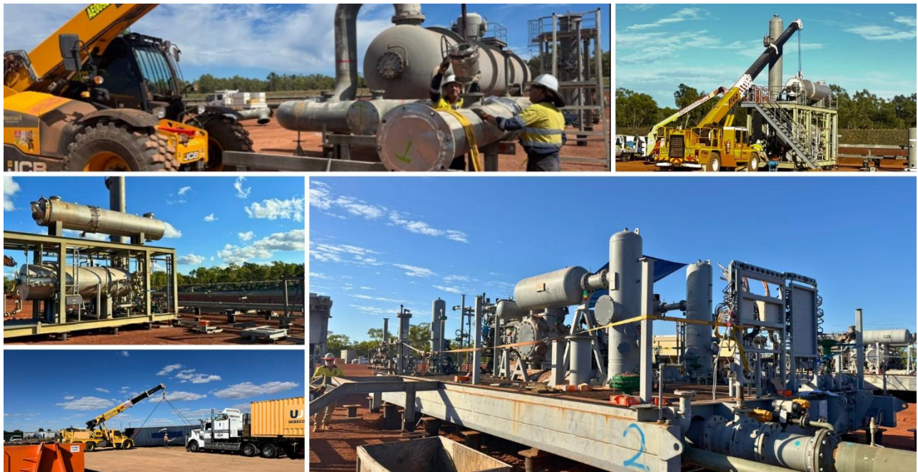
Construction of the Carpentaria Gas Plant
