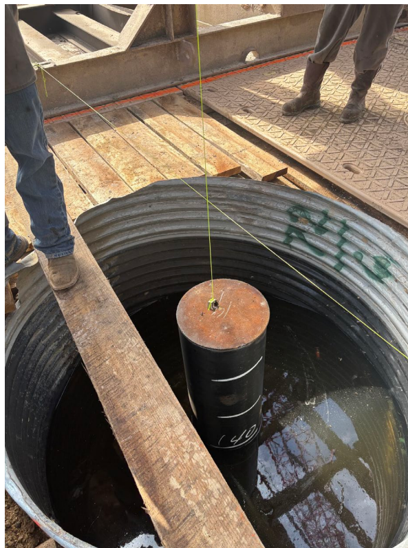
Figure 2: Conductor pipe installed and centred in the cellar ahead of final rig-up
