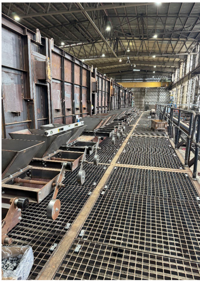
Quicklime piping and Reduction Furnace screw conveyor and platform installation progress
