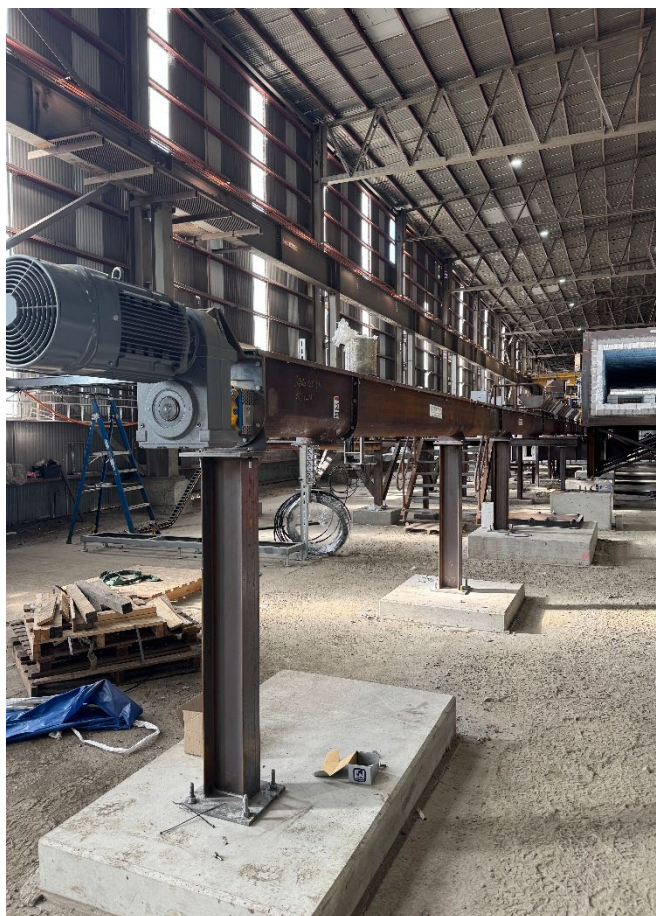
Quicklime piping and Reduction Furnace screw conveyor and platform installation progress
