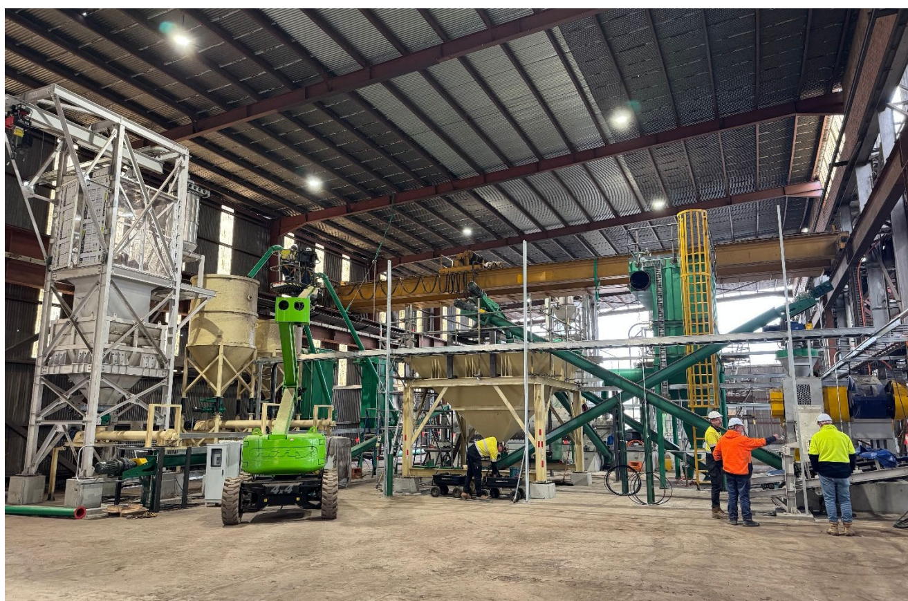
Briquetting area SMP installation progress
