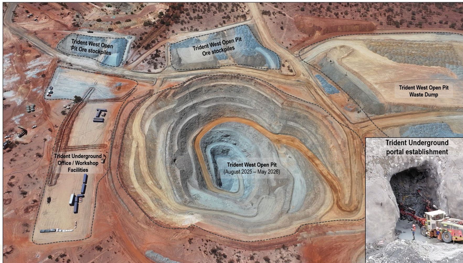
Figure 2: Completed Trident open pit. Inset shows commencement of portal establishment.
