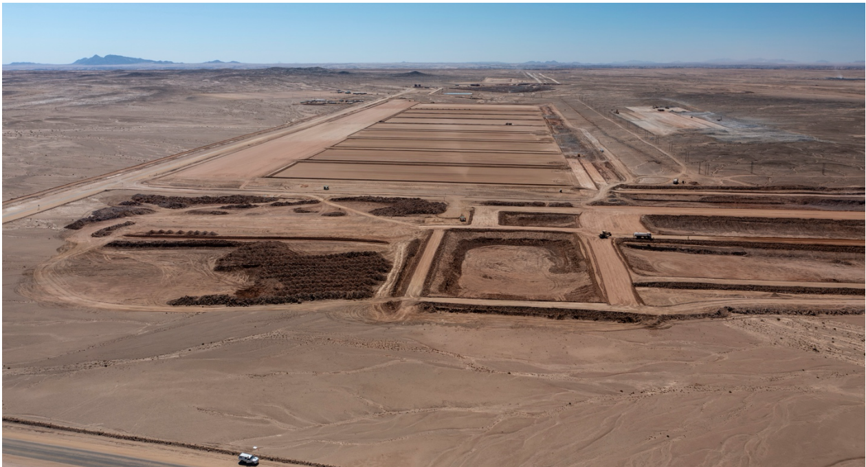
Figure 1: In addition to heap leach pad earthworks, works have continued on the wet plant terraces and solution ponds.
