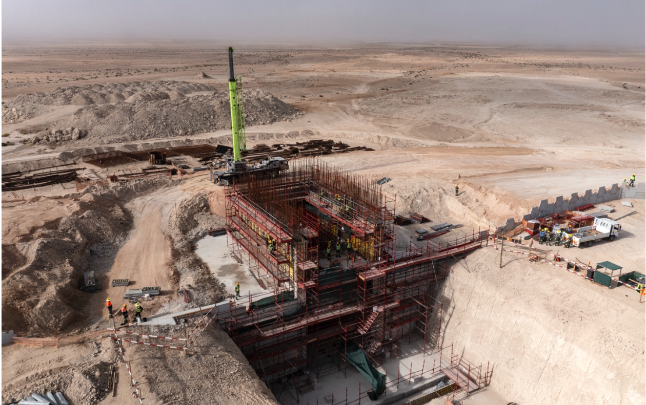
Figure 2: Primary crusher building structural concrete is now progressing above ground level.
