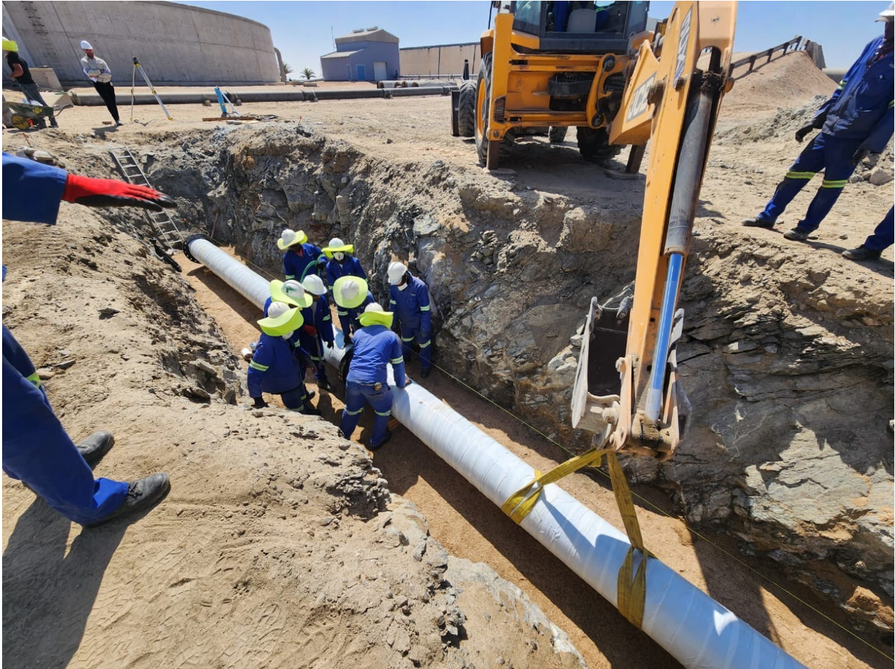
Figure 7: Underground pipe for the permanent water pipeline has been laid and backfilling is in progress.
