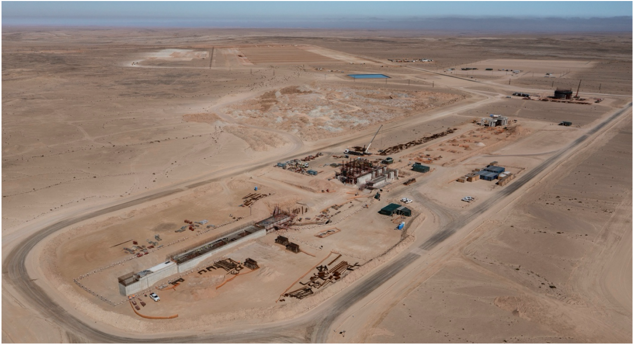
Figure 3: View of the dry crushing circuit. L-R Stockpile tunnel, secondary/tertiary crushing, secondary/tertiary screening, fine ore silo.
