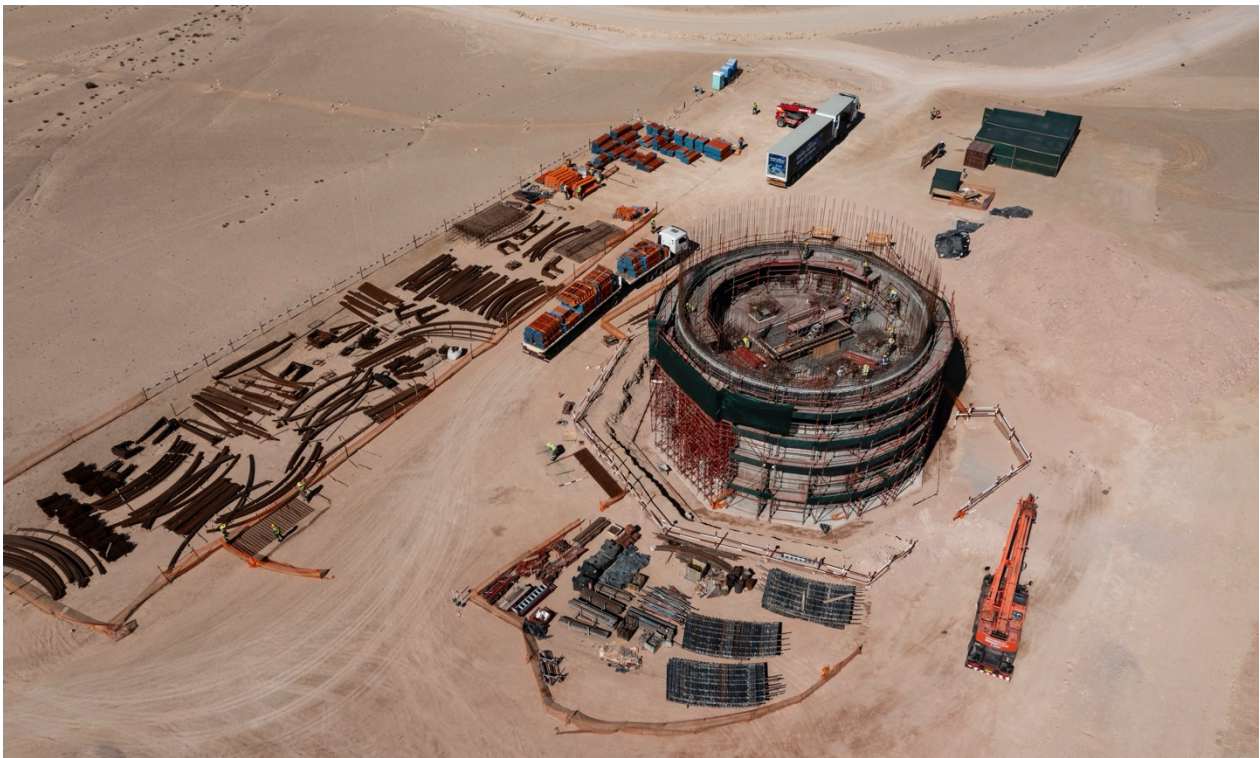
Figure 4: Aerial view of the fine ore silo which now stands approximately 36 metres above the ground.
