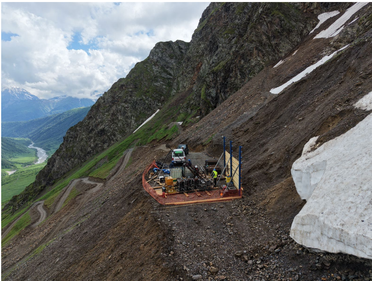
Figure 1 Drill rig on platform at Zopkhito
