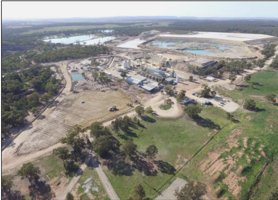
Figure 3: Mineral Hill Processing Plant and overview.
