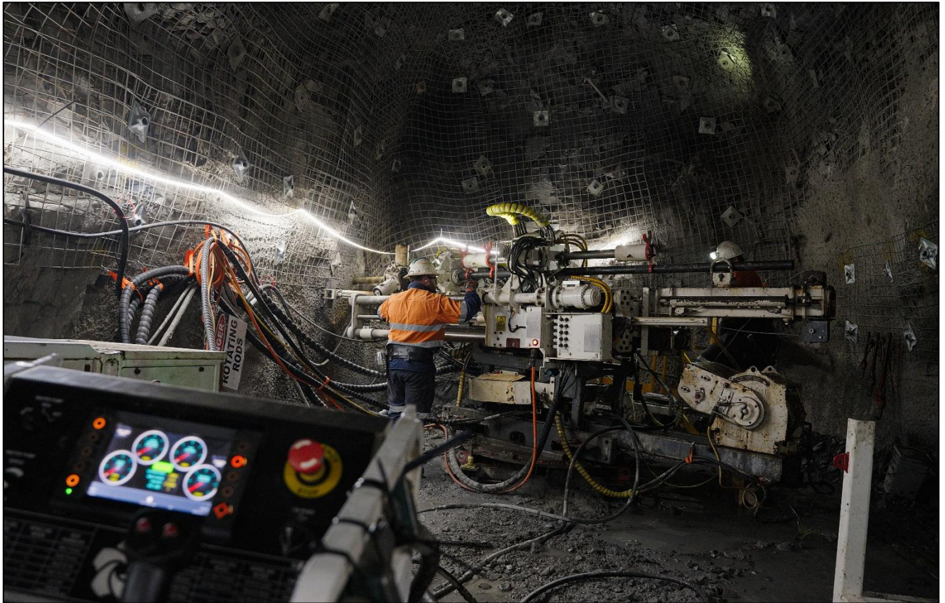
Figure 5: Current underground drilling.
