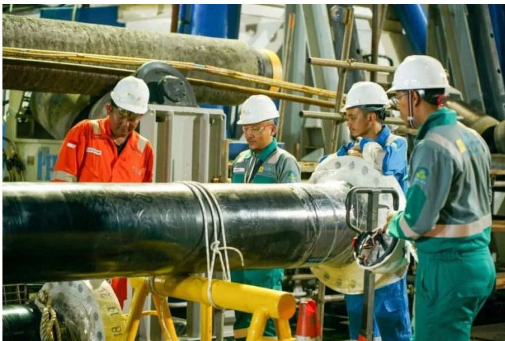
PLN EPI Project Experts carefully check the preparation of hot tap and tie-in works (ANTARA/HO-PLN EPI)
