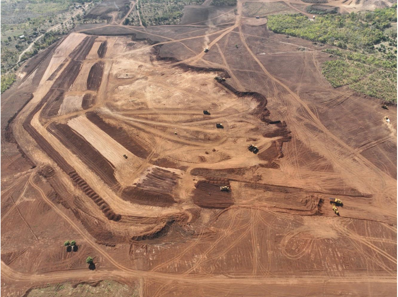
Picture 8. Kangankunde Tailings Storage Facility Progress
