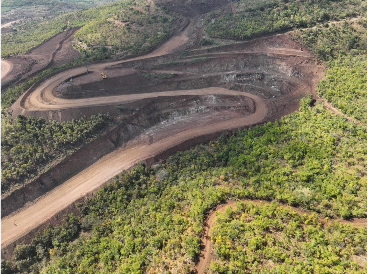
Picture 4. Completed haul road providing access to the Stage 1 pit area
