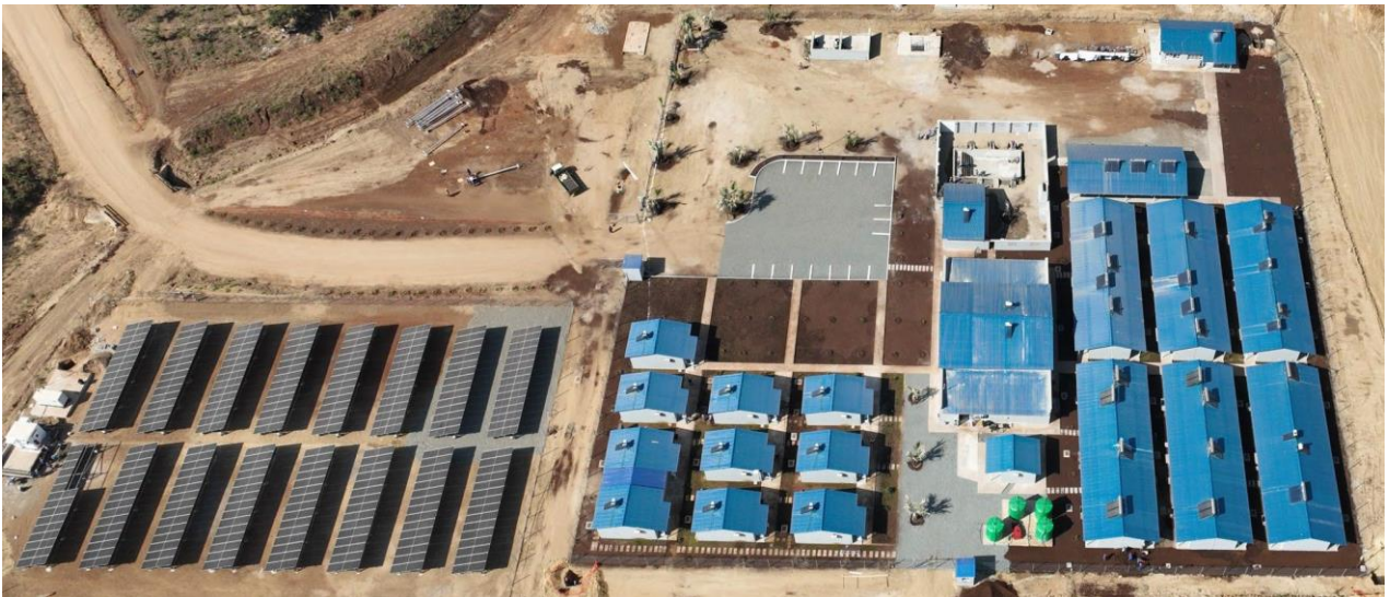
Picture 14: Kangankunde Timpe 90-personnel accommodation camp.
