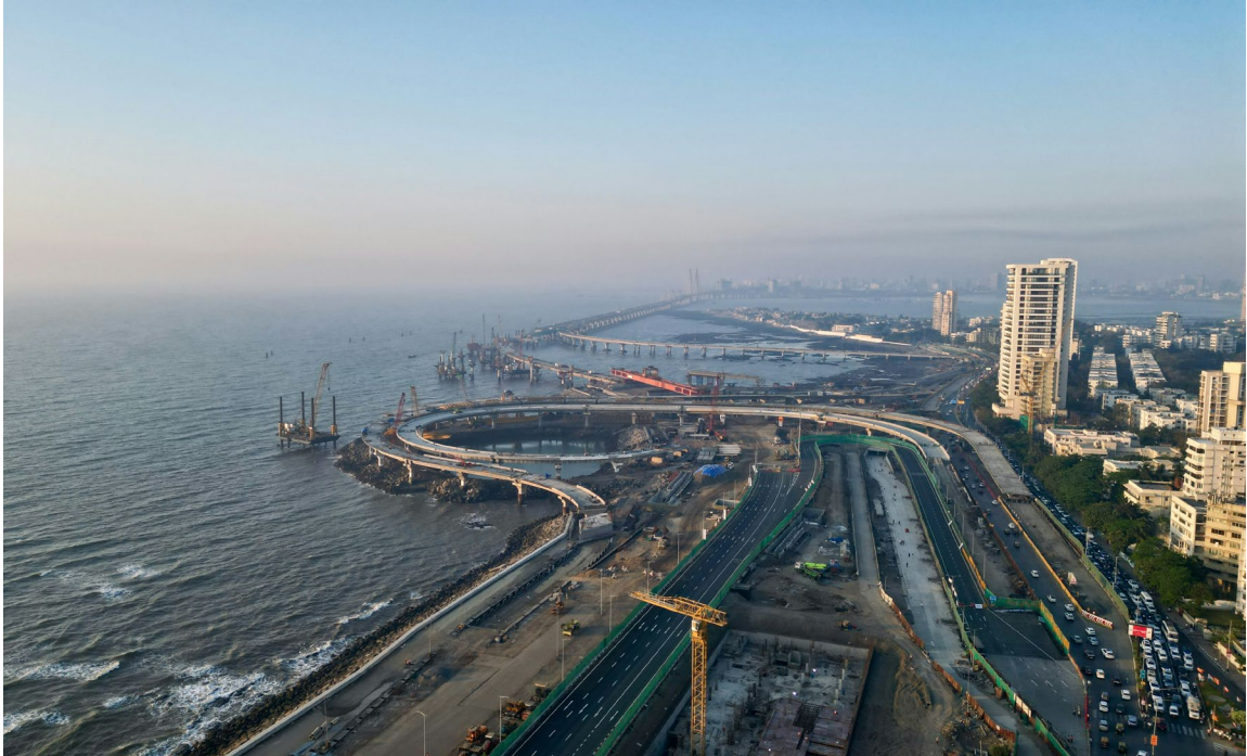
Photo 4. Road construction in India. Not associated with Eden’s recent trials.
