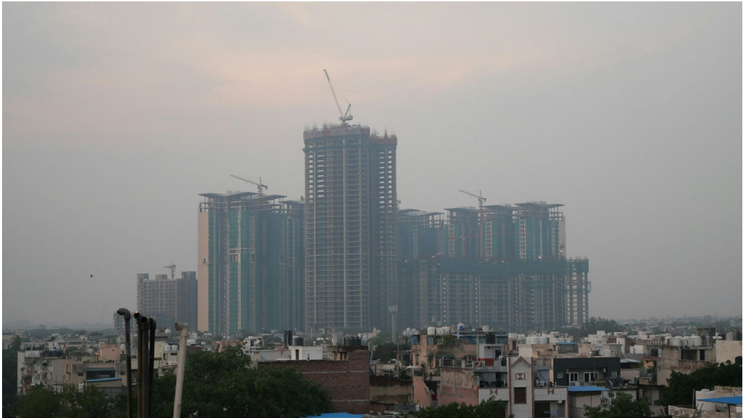
Photo 1. Indian high rise apartment project, not necessarily involving Eden's trials
