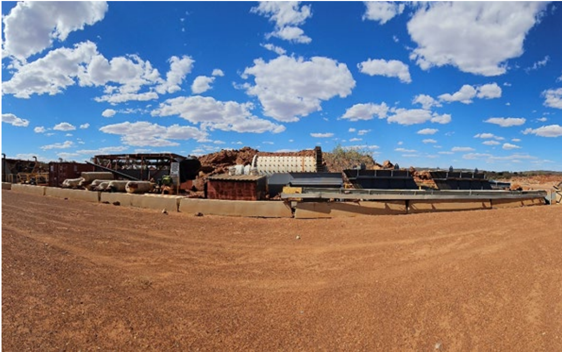
Figure 1: Ball Mill and associated plant
