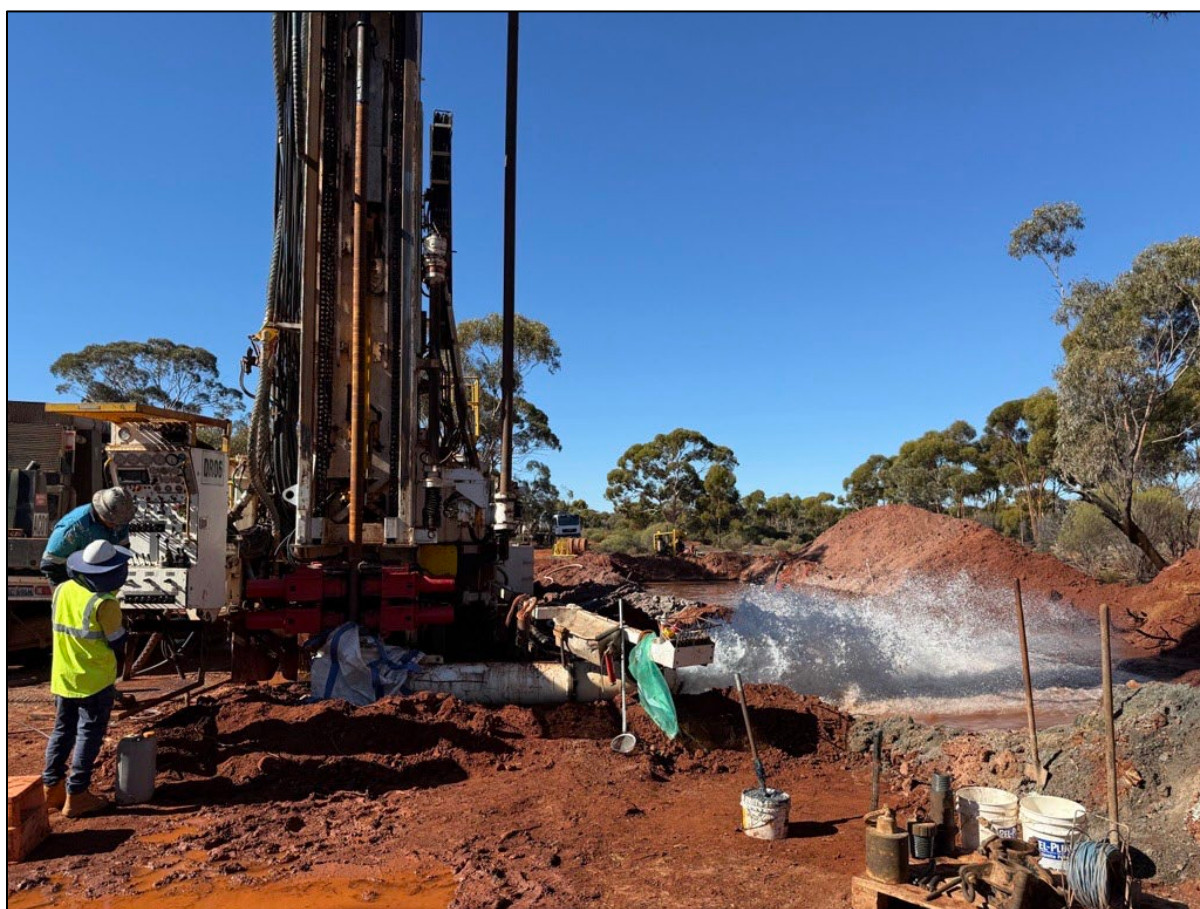
Figure 2: Water bore airlift testing
