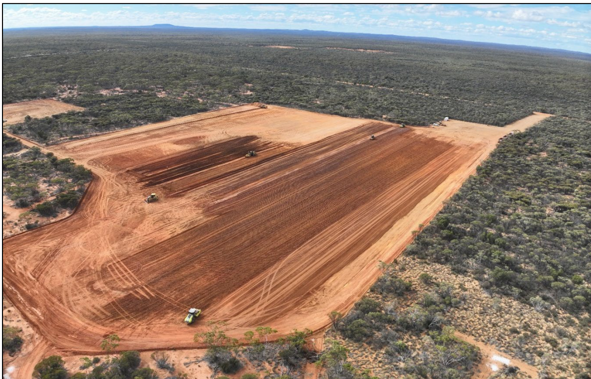
Figure 1: Village site preparation and bulk earthworks
