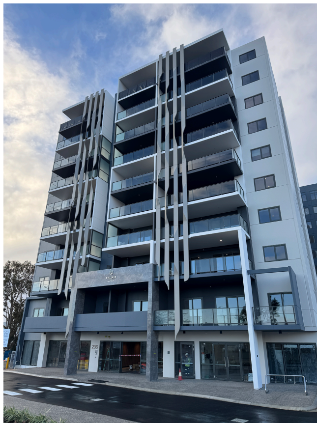
Figure 1. Bel-Air Apartments site photo, Belmont
