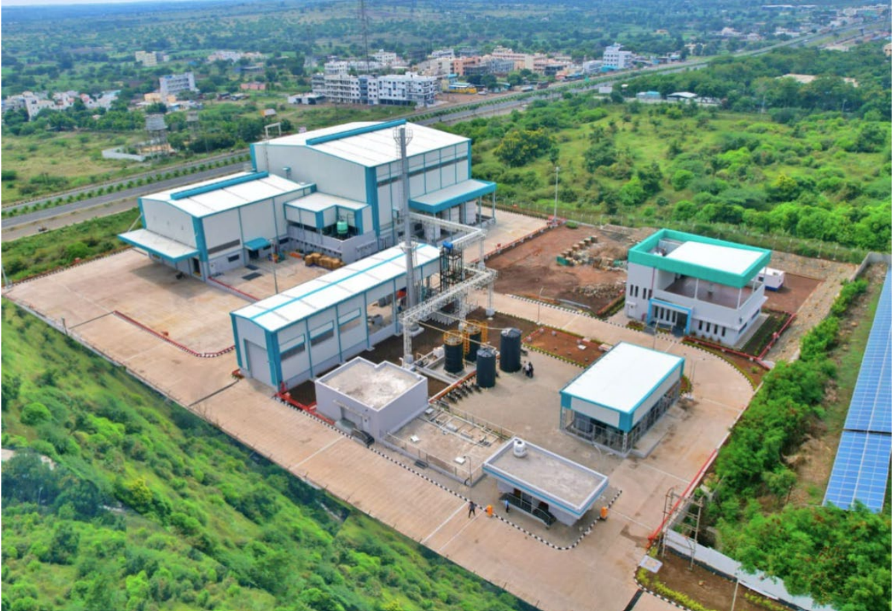
Expandable Graphite JV Facility near Pune, India
