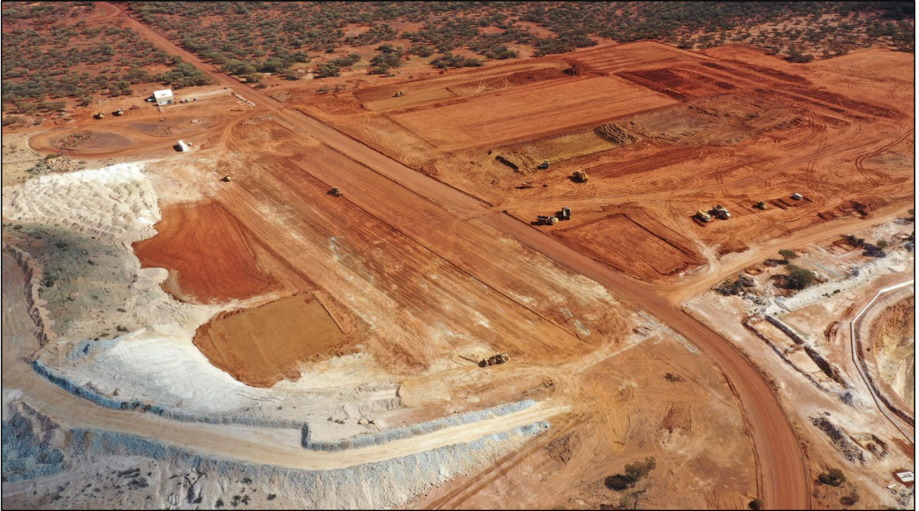
Figure 6 – Processing plant bulk earthworks nearing completion
