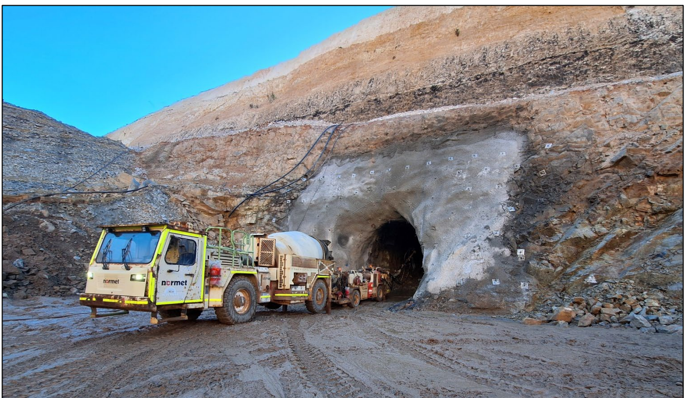
Figure 1 – Stripping at the Youanmi Decline
