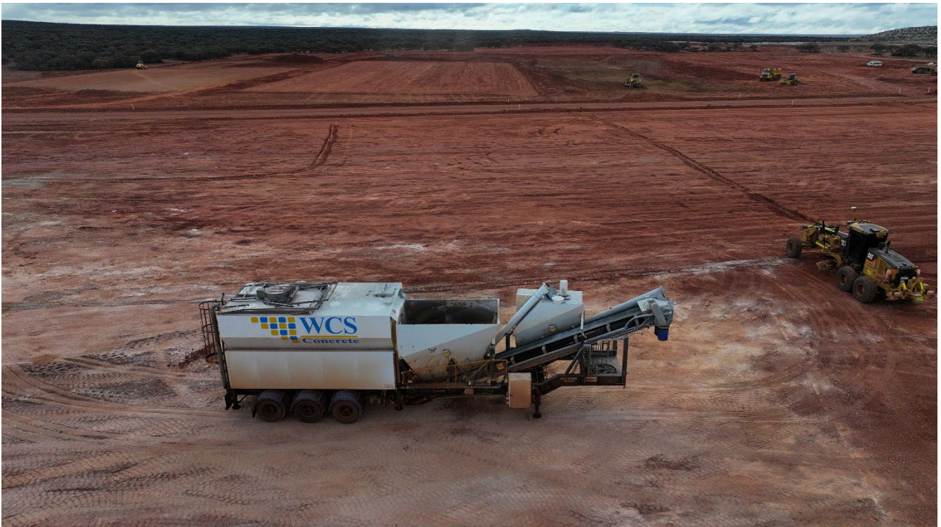
Figure 7 – Interquip Mobilisation underway
