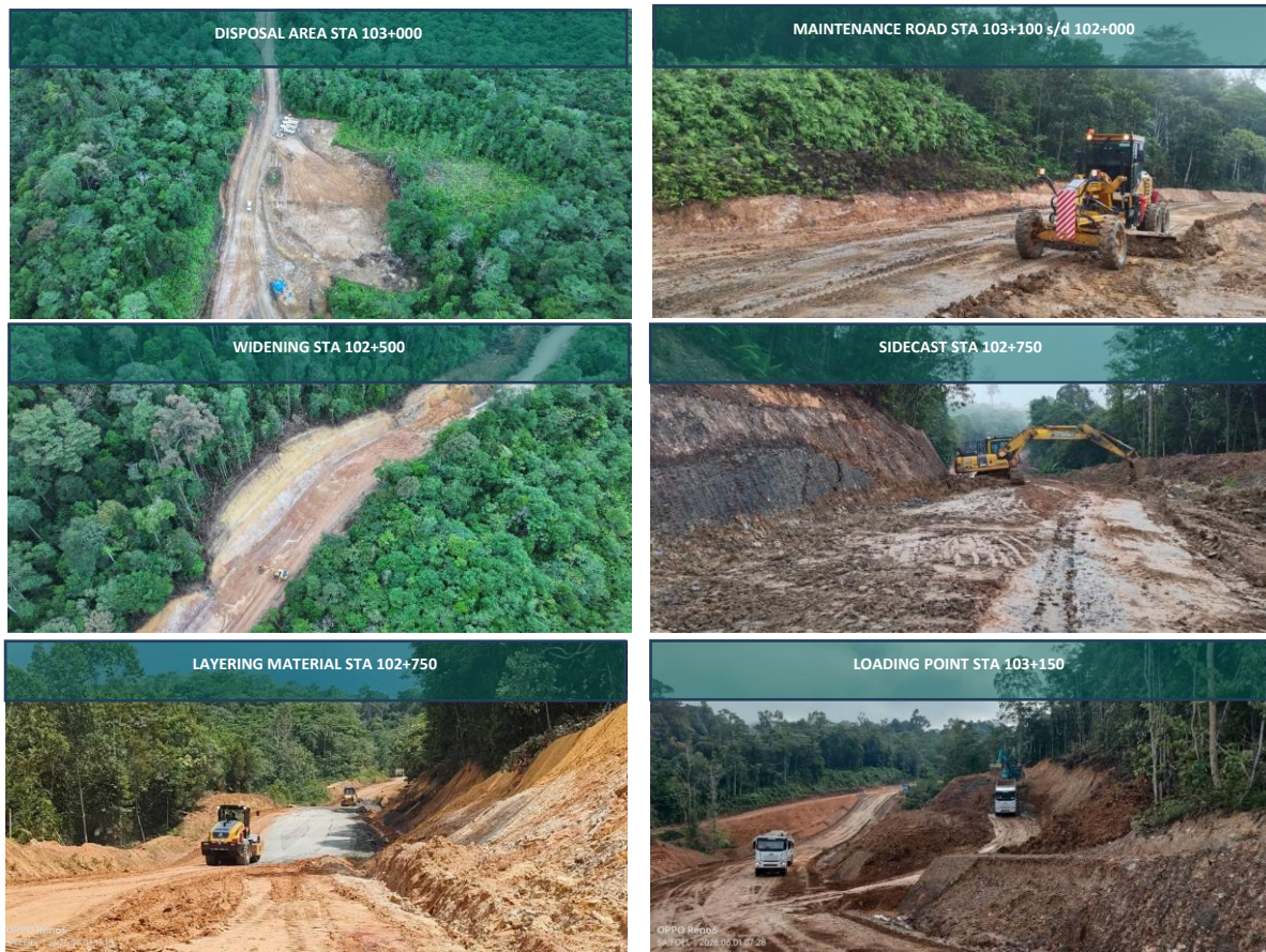
Segment B4 (STA 104+575 – STA 96+250) progress
