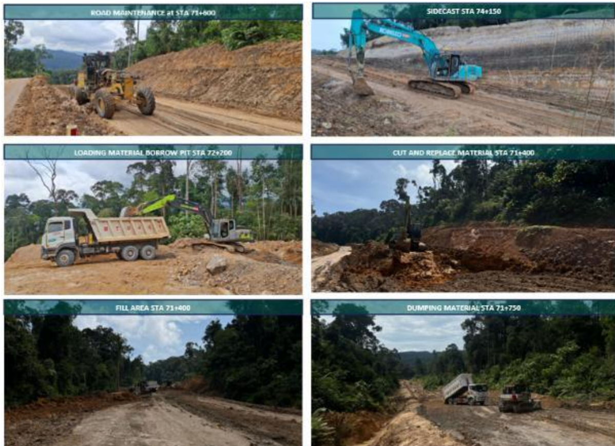
Segment B2 (STA 85+875 – STA 69+775) progress
