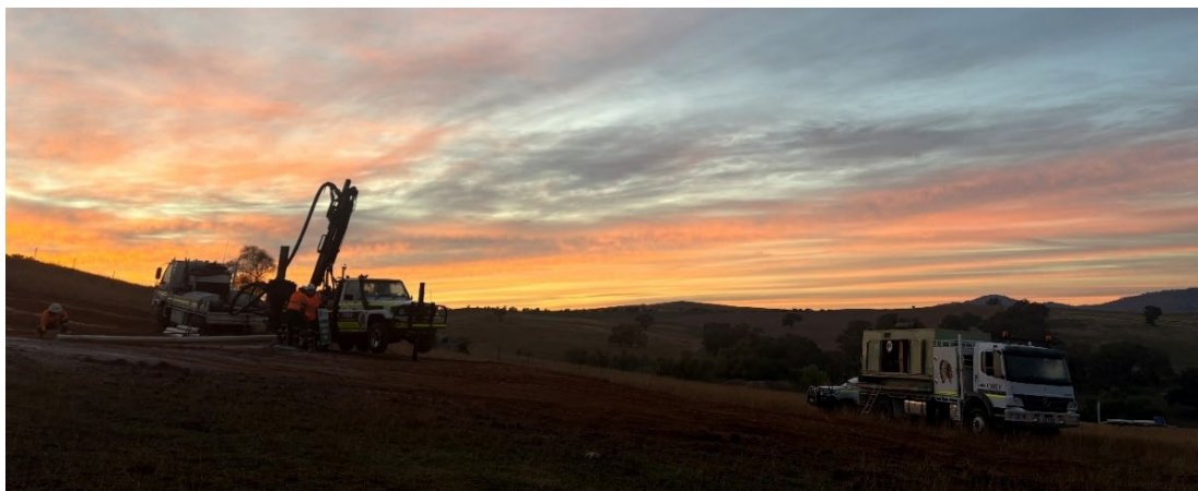
Figure 1. Drilling commenced at the McMahons Reef Prospect, Harden, NSW.
