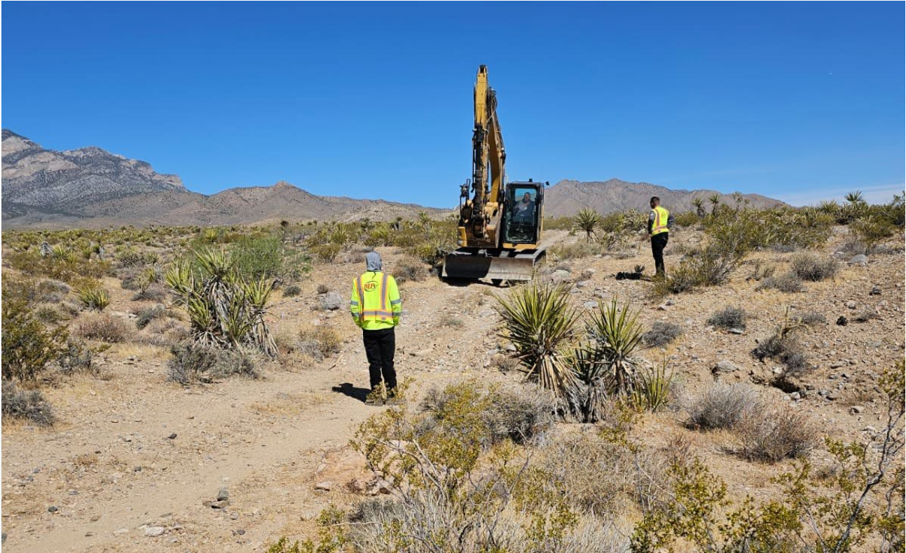
Figure 5: Access track upgrade works at Desert Star
