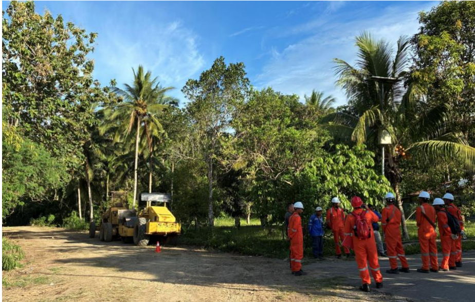
Figure 1: Road access clearing operations
