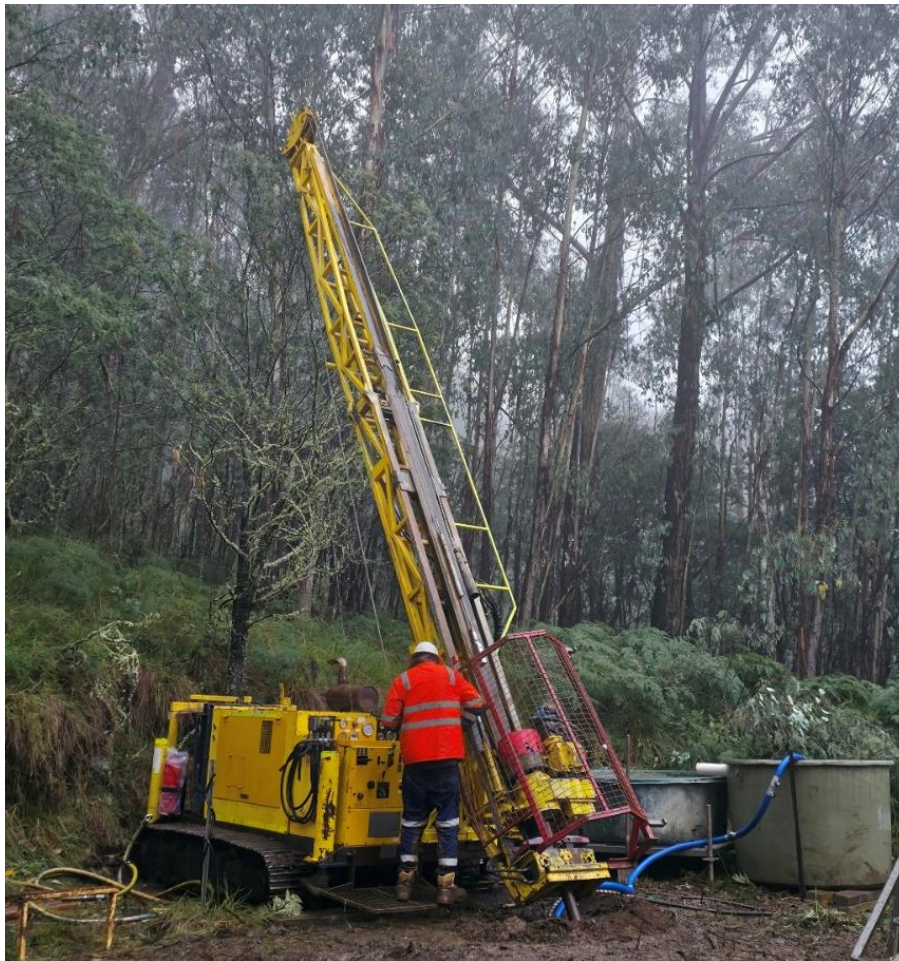
Figure 1: Cortech Rig drilling 25SSDH001
