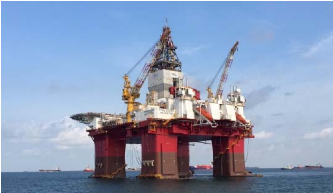
Photo 1: Transocean Equinox Semi-Submersible Mobile Offshore Drilling Unit
