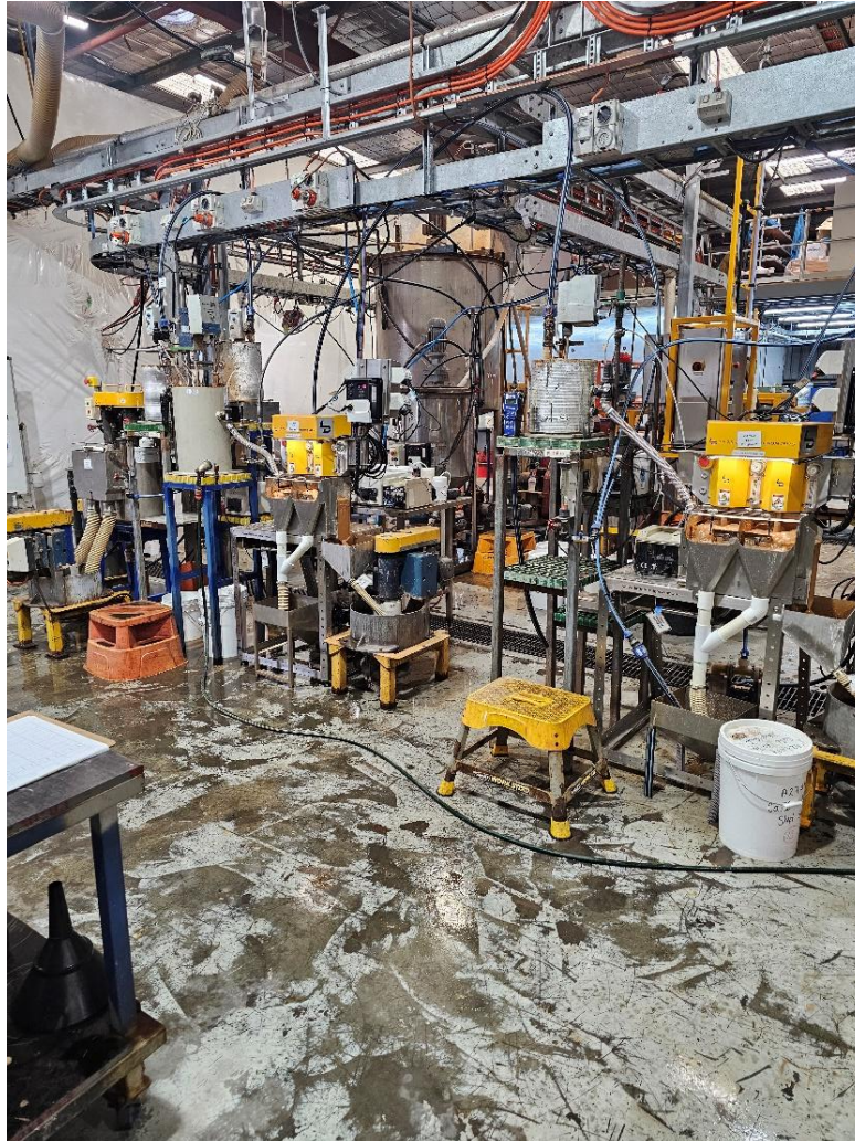
Figure 2: Rougher flotation setup with cyclone, surge tank, sulphide flotation cells and fluorite flotation cells
