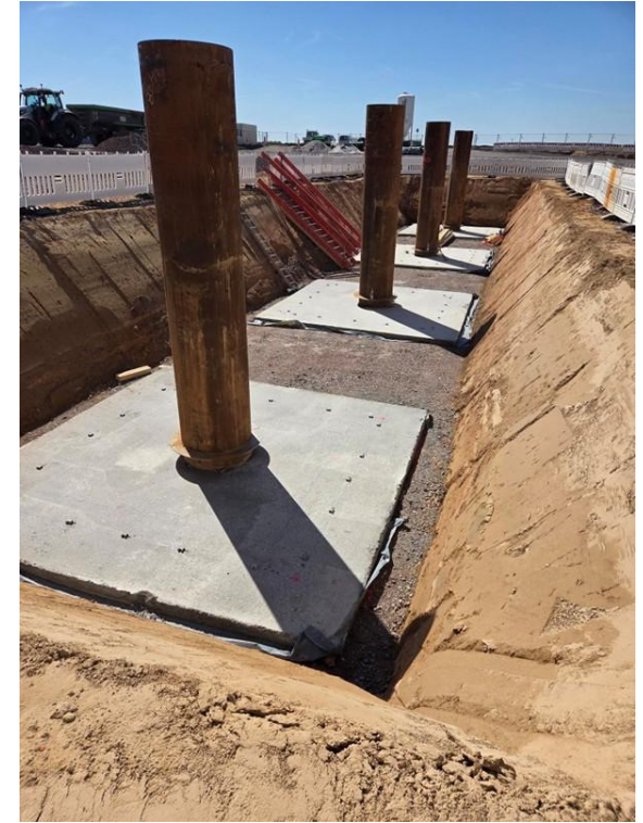
From left to right - relocation of the 110kV overhead power lines, underground power cables to replace overhead and drainage works at the integrated geothermal and lithium extraction site near Landau. Far right - concrete cellars for the new well pad at one of the new production well sites.
