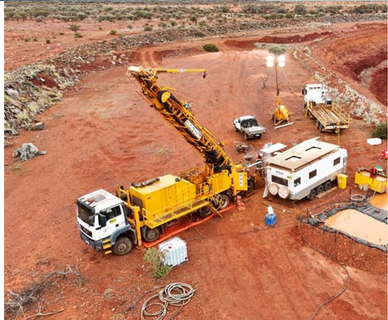
DDH1 Drilling rig on site at Western Queen South
