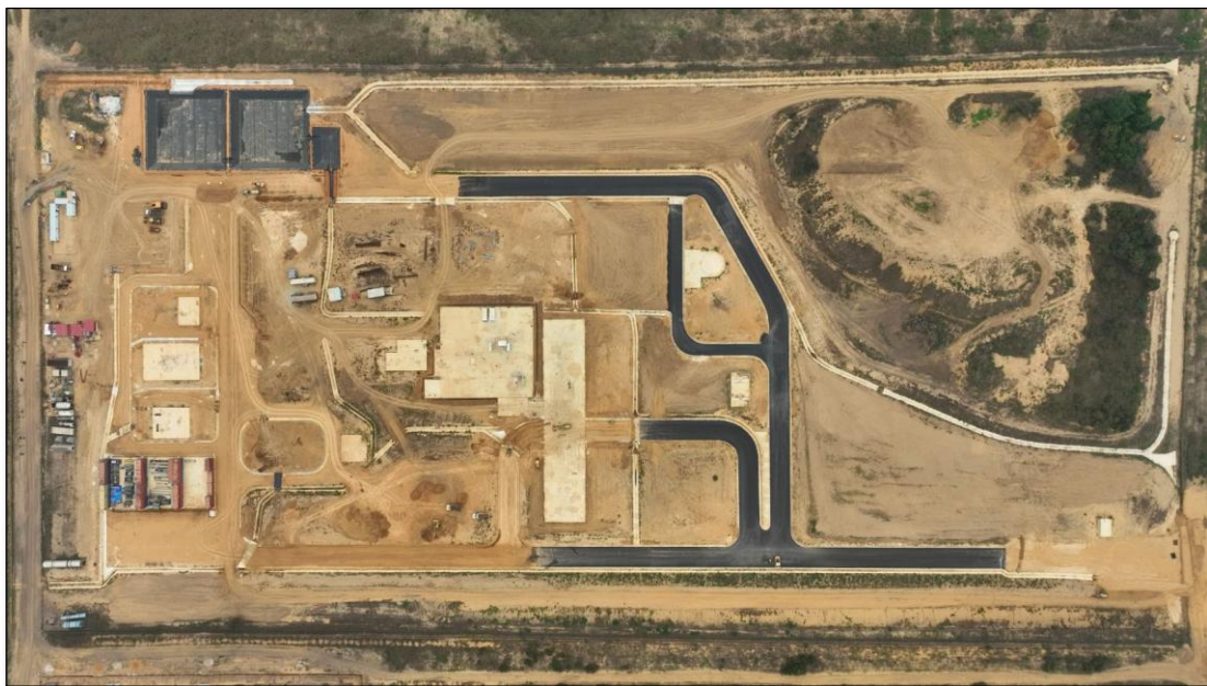
Figure 2 – Cabinda Phosphate Fertilizer Project, located in Cabinda Angola, with Phase 1 construction works now completed.
