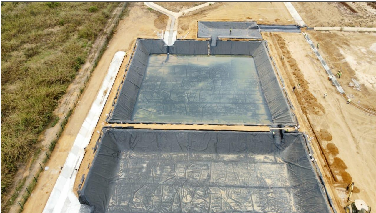
Figure 4 - Cabinda Phosphate Fertilizer Project, water run-off settling ponds.
