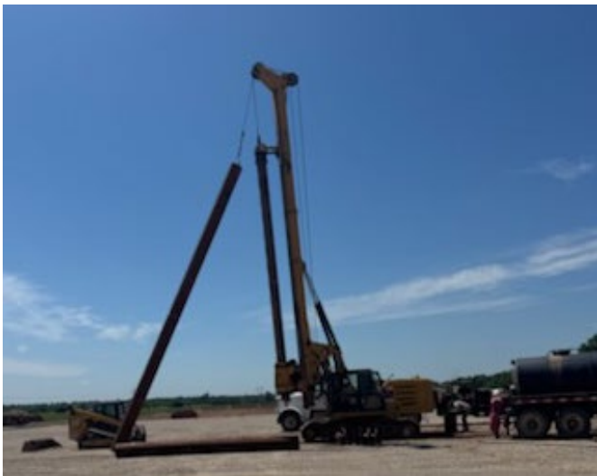
Conductor set for the Sabres and Whalers wells at Brookside's SWISH AOI two-well development pad
