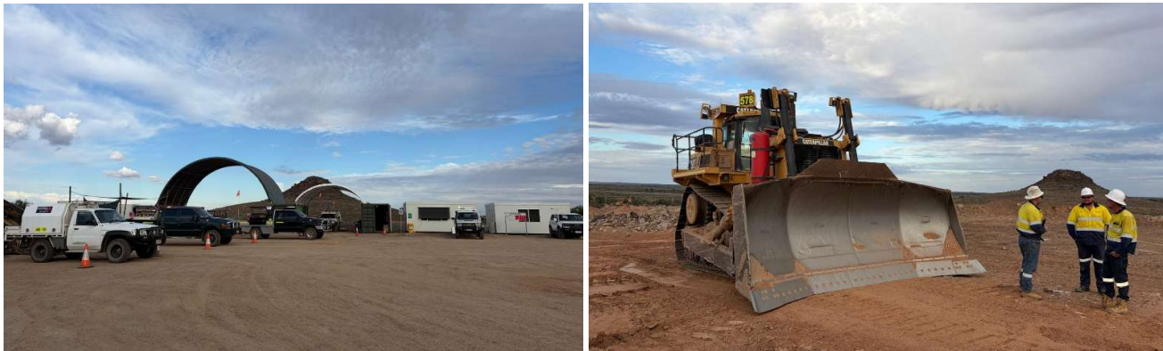
Figure 3 – Newly established administrative offices & ROM Pad clearing activities
