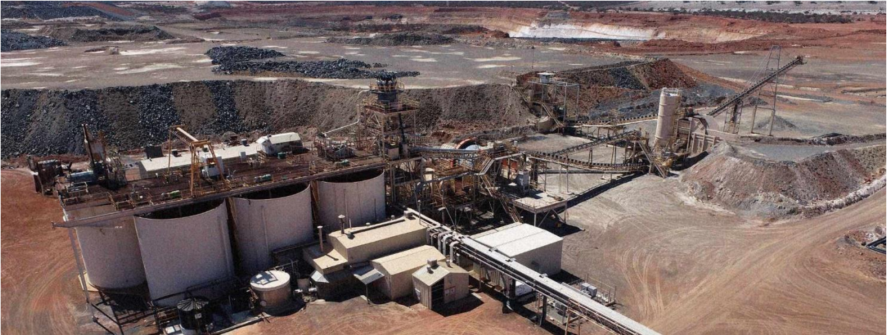
Figure 6. Kirkalocka Plant and ROM Pad with Kirkalocka open pit in the background (operated by Gylden Resources Pty Ltd)
