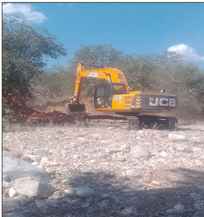
Figure 1 - Drill Readiness Works at Chalkos
