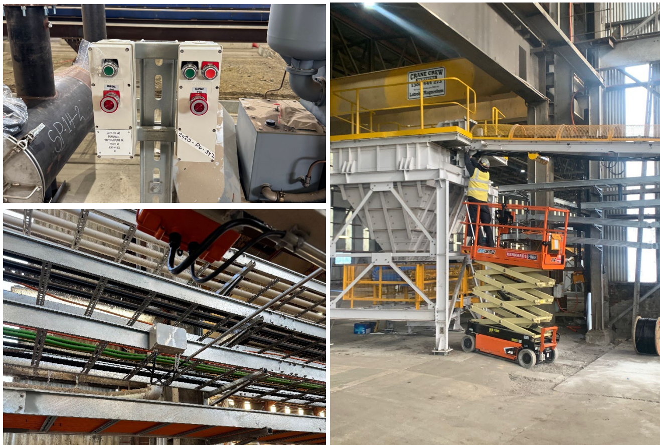
E&I activities in Reduction Furnace and Briquetting areas
