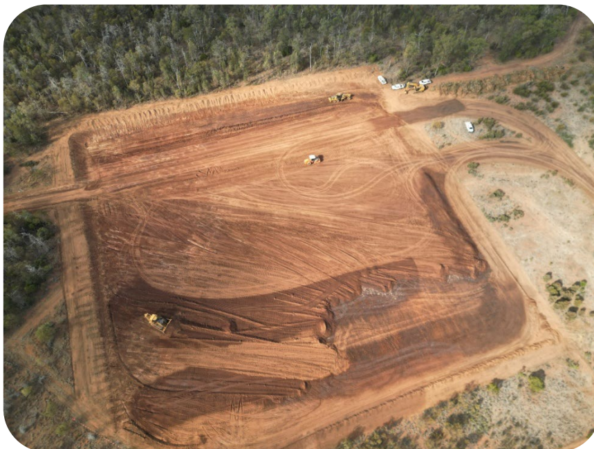
Figure 1: Well-pad preparation
