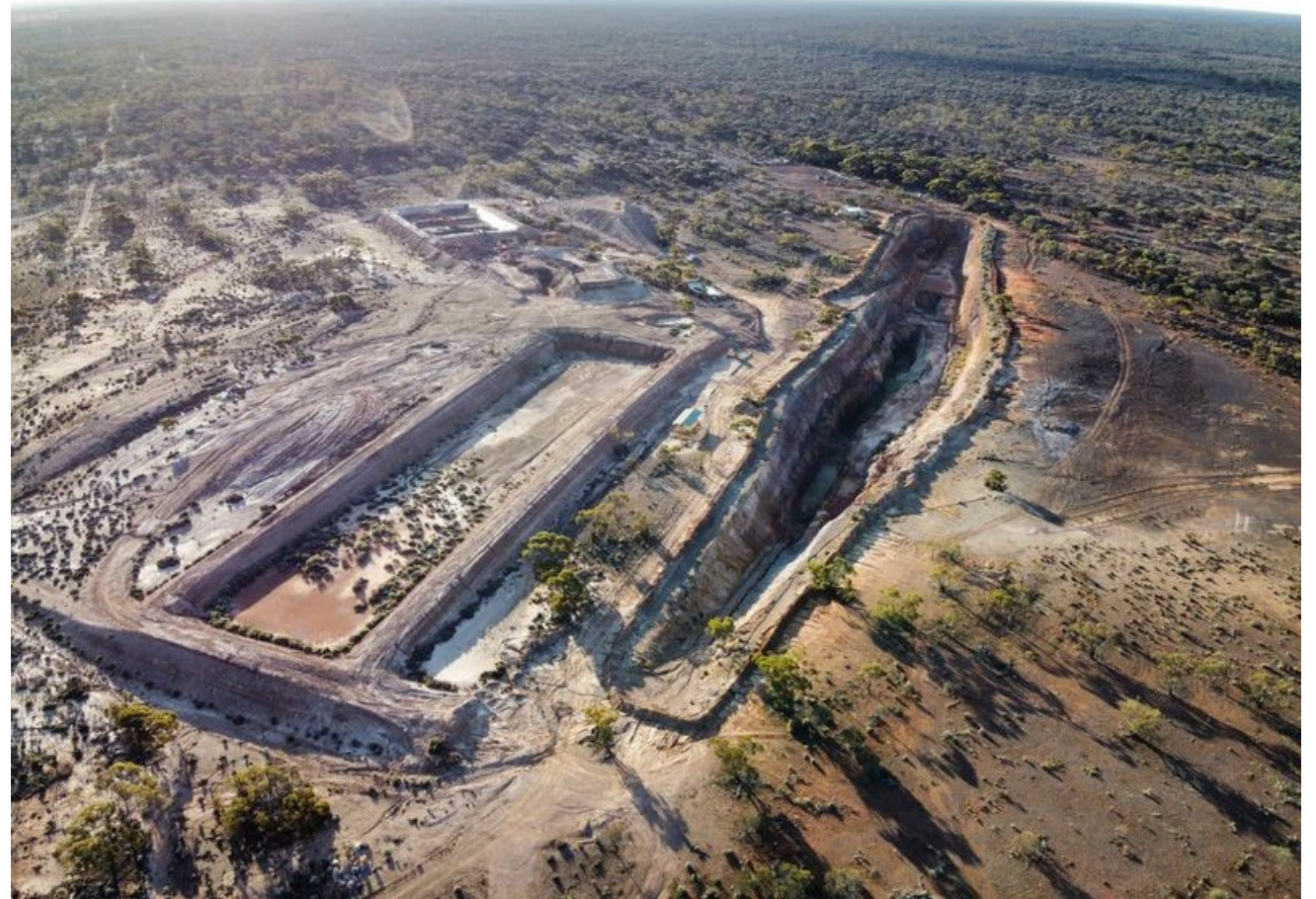
Drone photo of Zelica Project looking NNW showing pre-stripped open pit (approx. 300m long and 10-25m deep) and pre-constructed vat leach ponds (pic taken August 2025)
