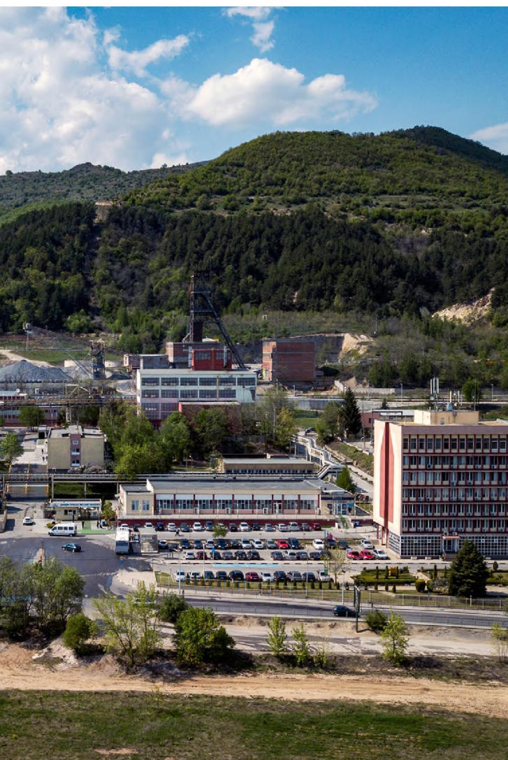
Surface facilities at the Chelopech mine site
