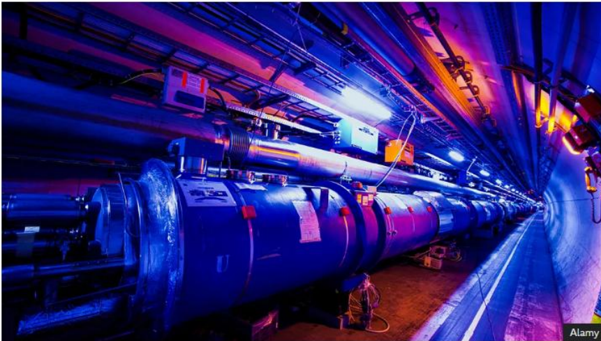
Liquid helium is used to cool the superconducting magnets at facilities such as the Large Hadron Collider (Credit: Alamy)
