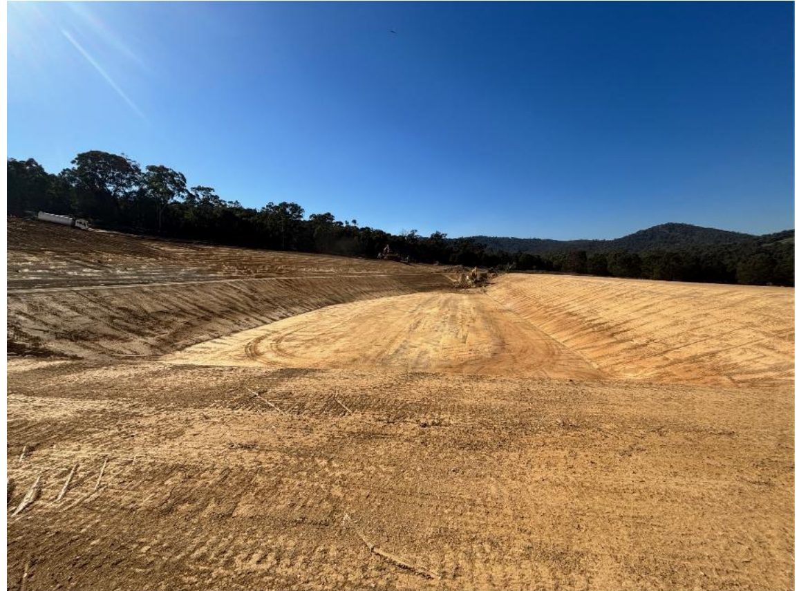
17 megalitre water dam preparation looking east, note excavator for scale
