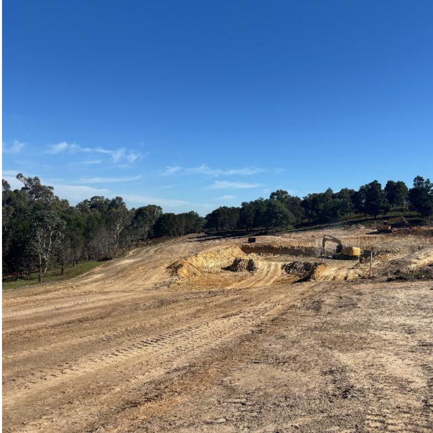
Box cut earthworks
