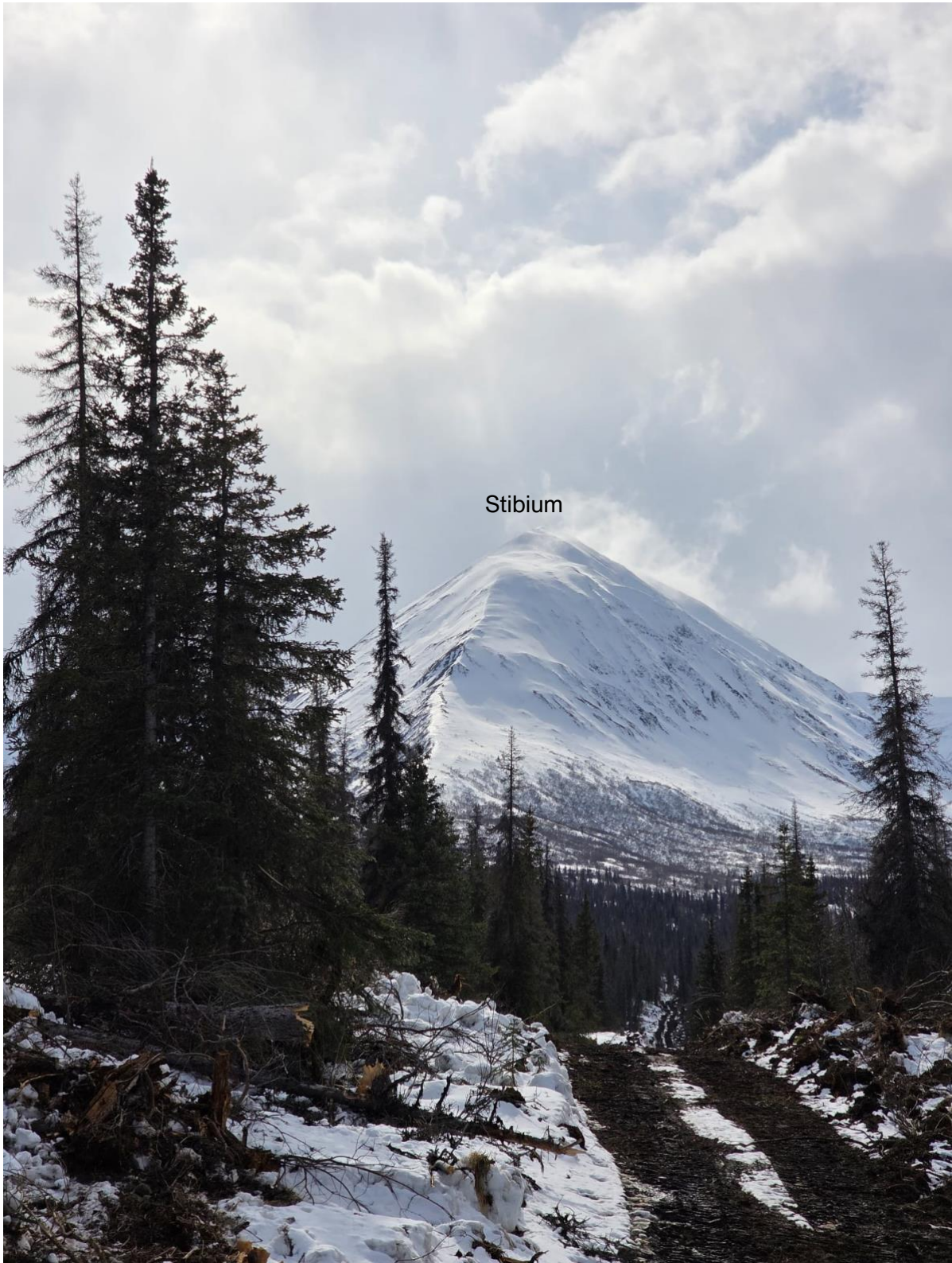
Figure 4. Construction of the Stibium access trail with the Stibium antimony-gold prospect visible in the background.
