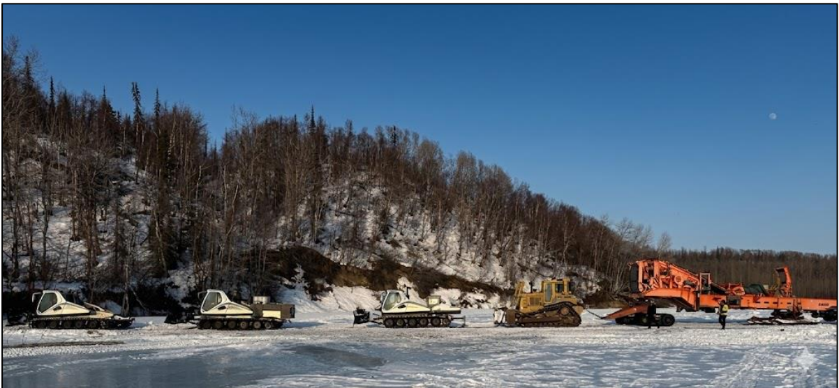
Figure 3. Snow road operations showing three snowcats and a D7 bulldozer linked together, combining 1,825 horsepower about to haul the screen plant up the steepest trail section
