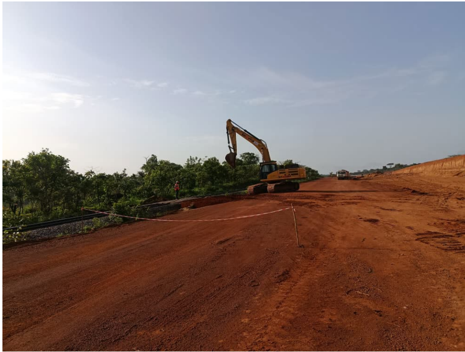
Image 2: Site works at IRF
