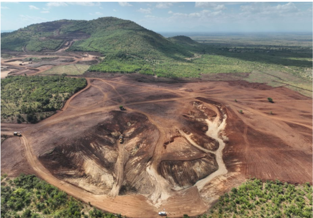
Picture 2. Topsoil Removal at TSF
