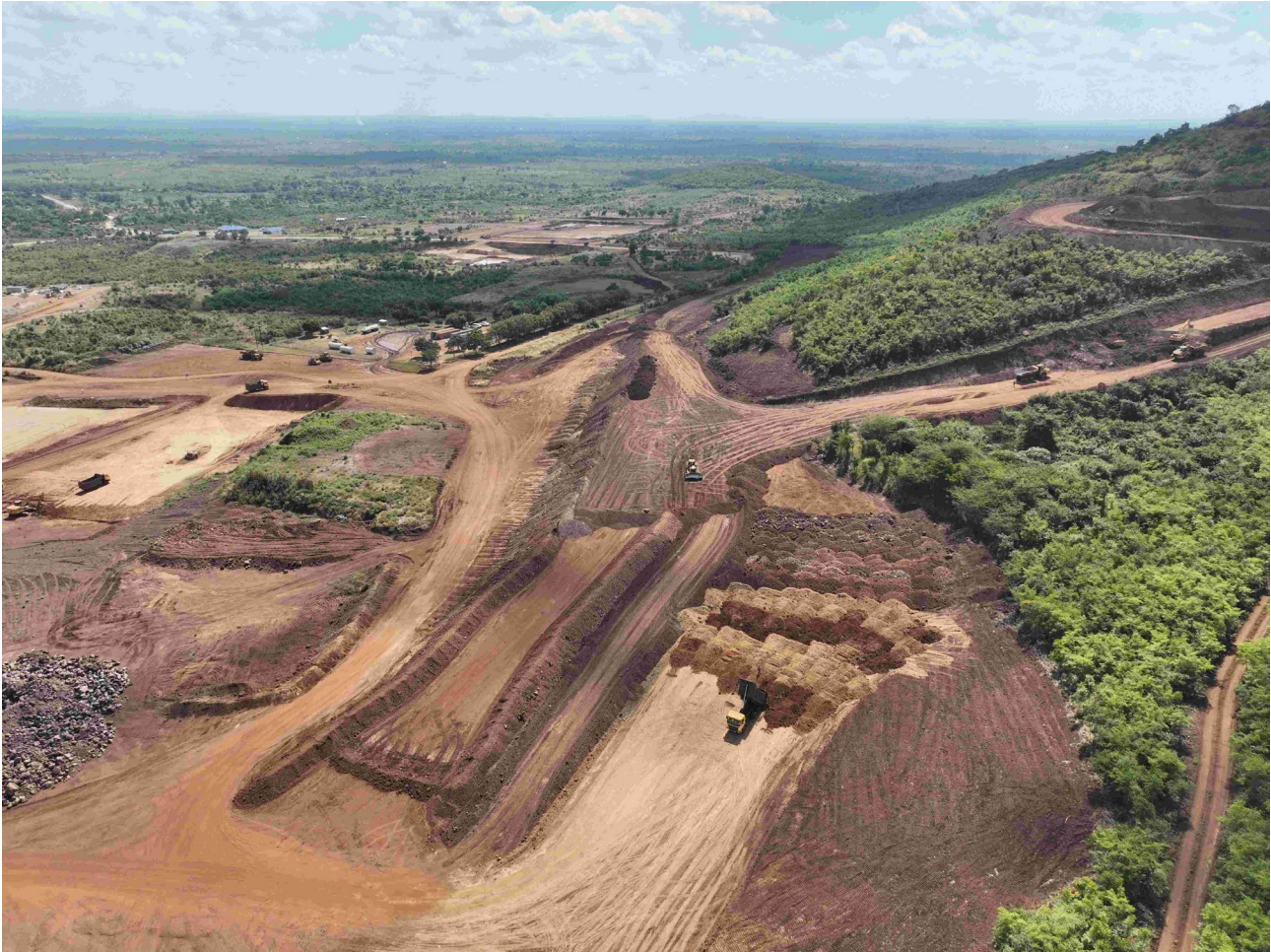
Picture 9. ROM pad and skyway expansion in progress
