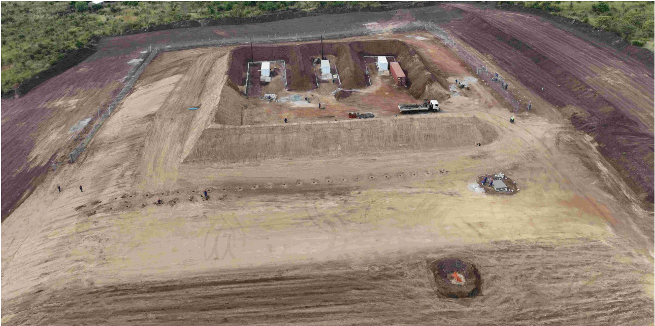
Picture 7. Explosive magazine and dual fence
