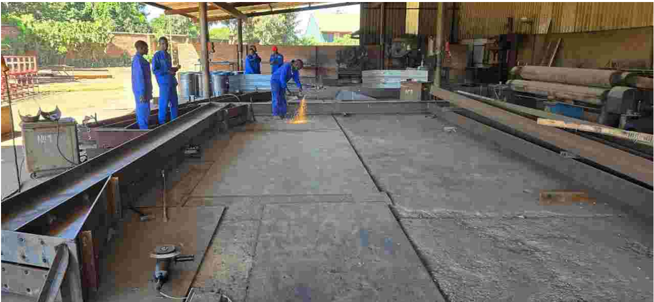
Picture 6. Offsite steel fabrication works
