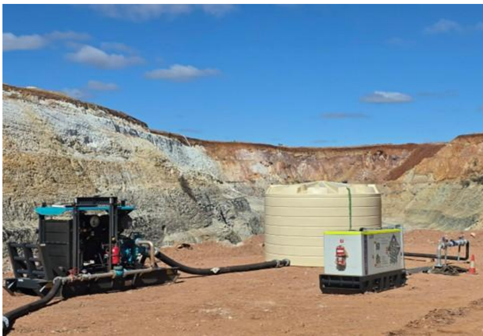
Figure 2 – Youanmi Main initial UG dewatering setup
