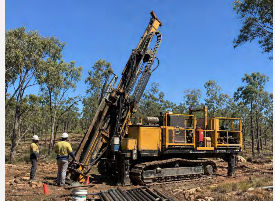
Track mounted drill rig
