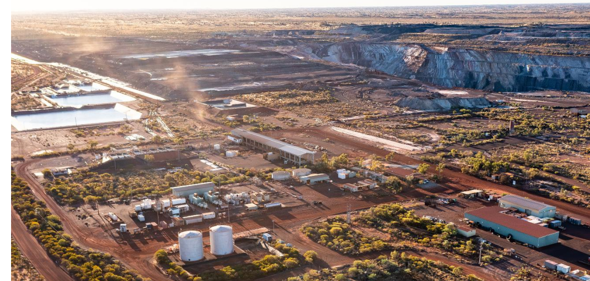
25,000 TONNE CAPACITY SXEW PLANT
