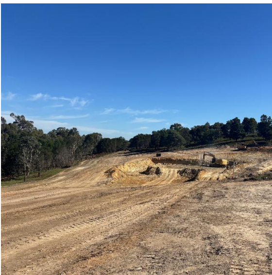
Figure 1. Box cut earthworks, 30 April 2026.
