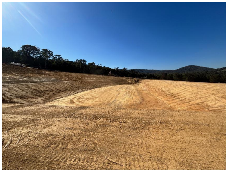
Figure 2. 17 megalitre water dam preparation looking east, note excavator for scale 30 April 2026.
